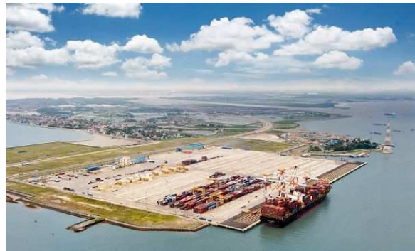
General View of Lach Huyen International Gateway Port (Opening in 2018)
