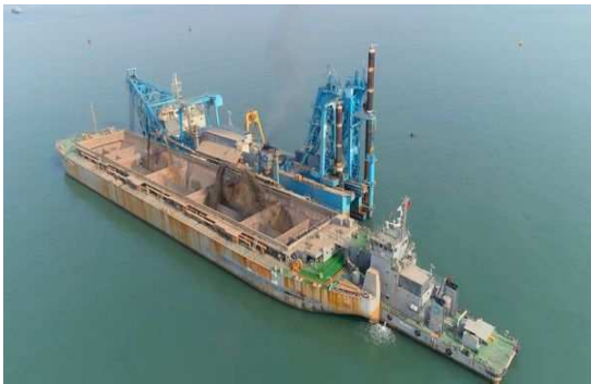
View of Dredging for Navigation Channel by Own Dredging Fleets (Package 9)
