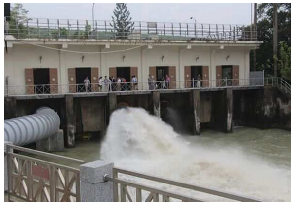
Special Discharge of Water from the Former Outlet
