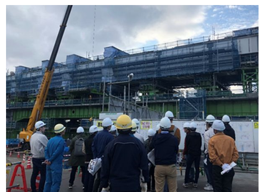
Students Learned about the Viaduct
