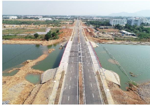
Photo 2 New bridge that goes across the reservoir
