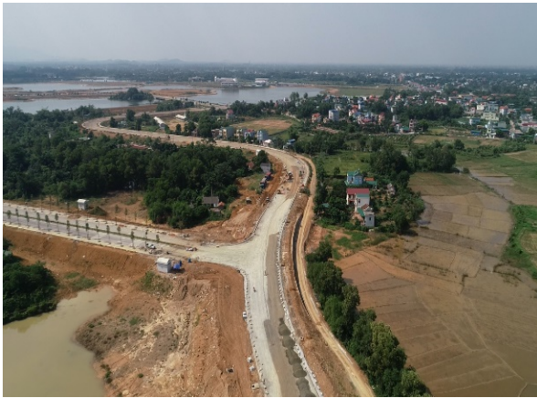
Photo 1 Construction of new road
