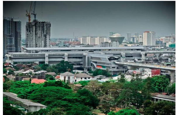
Tao Poon Station – Intersection of MRT Purple Line and Blue Line
