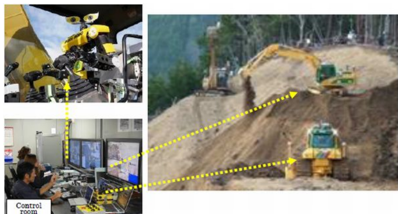
Unmanned construction technology used in disaster recovery
