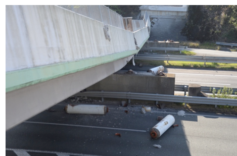
Photo 1: Collapse of Furo Overbridge onto the Kyushu Expressway
