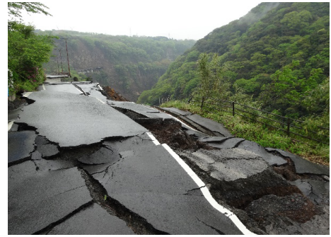
Photo 5: Damage and collapse of the access road connected to the Aso Choyo Ohashi Bridge
