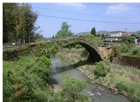
Photo 2: Deformation of the upper part of the stone wall of Tsujunkyo Bridge (above) and collapsed masonry wall of Shimotsuru Bridge (Uki City) (below)
