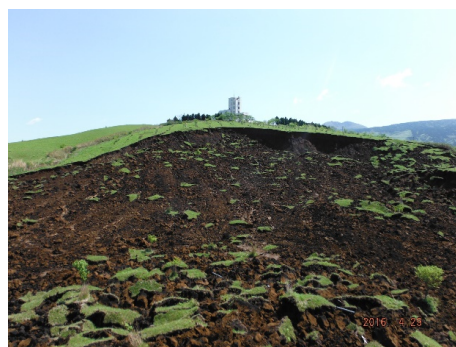
Photo 4: Landslide that occurred on a gently inclined slope
