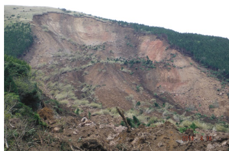
Photo 3: Large-scale slope failure that caused the collapse of Aso-Ohashi Bridge
