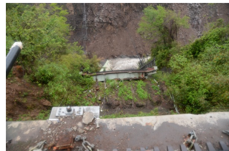
Photo 3: Collapse of Aso-Ohashi Bridge due to slope failure
