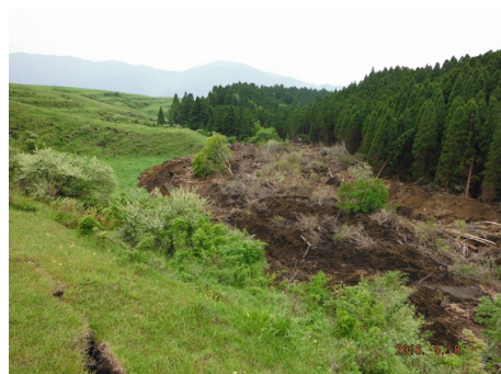
Photo 11: Collapsed sediment blocked the outlet of a valley, downstream of which is the Sannodani River.
