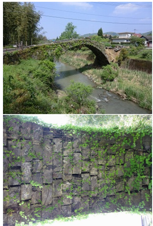
Photo 5: Collapse status of the masonry wall of Shimotsuru Bridge (Uki City) and gaps that developed between the arch stones
