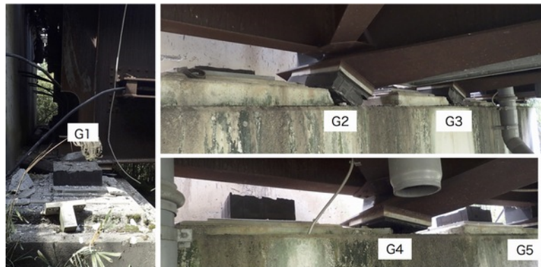
Photo 2: Abutment of Okirihata Bridge with broken rubber bearings
