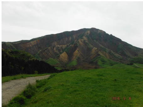
Photo 10: Surface failure on the south slope of Mt. Eboshidake
