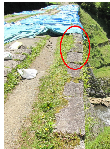
Photo 4: Deformation of the upper part of the stone wall of Tsujunkyo Bridge
