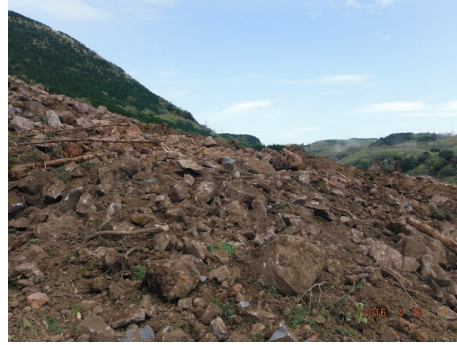
Photo 7: Collapsed sediment and rock mass deposited on gently inclined area
