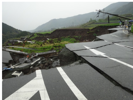
Photo 12: Collapse of the road leading to Aso Choyo Ohashi Bridge
