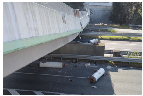
Photo 1: Collapse of Furyo Overbridge onto the Kyushu Expressway
