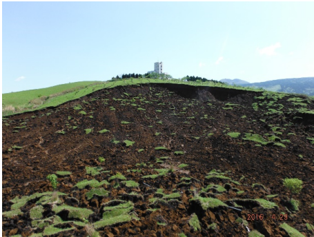
Photo 8: Surface failure that occurred on a gently inclined slope
