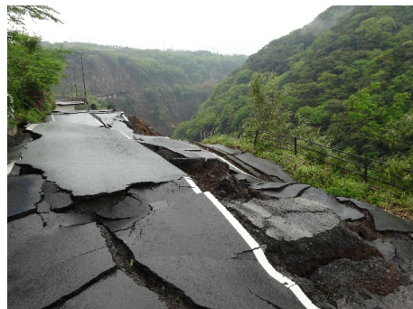
Photo 13: Damage and collapse of the access road connected to the Aso Choyo Ohashi Bridge
