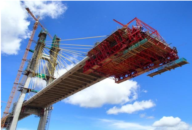
Photo 3. Balanced cantilever erection
