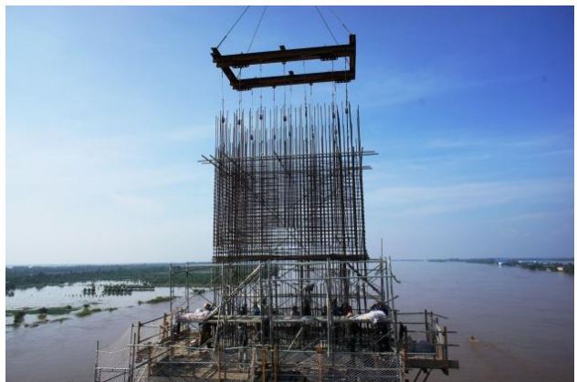
Photo 6. Erection of prefabricated rebar-cage
