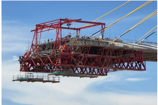
Photo 4. Underslung form traveller
