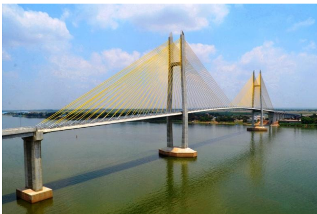
Photo 1. General view of main bridge
