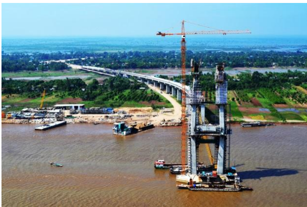
Photo 5. Construction of main towers
