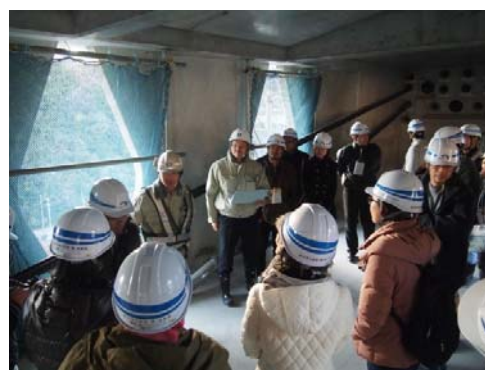
At the Akutagawa Bridge Work site
