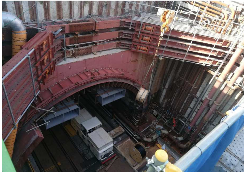
Picture 1.1. Image from the construction site of tunnel construction of the Haneda Airport
