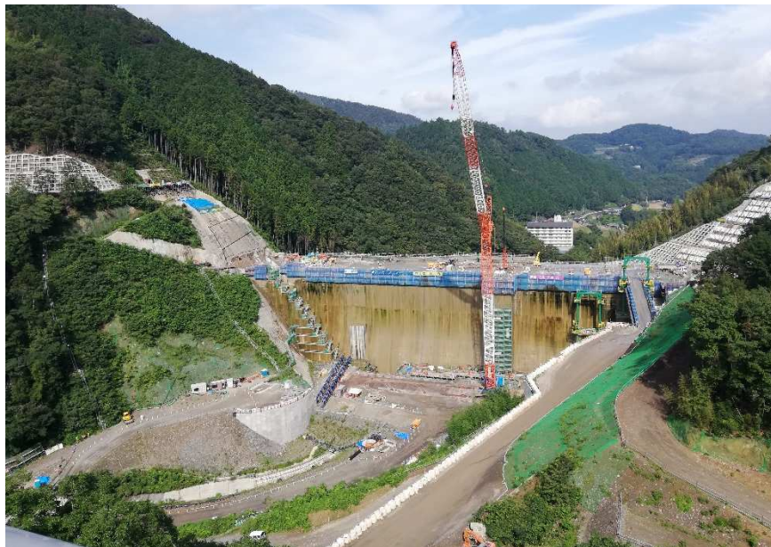
Picture 1.3. Kabagawa Dam construction site
