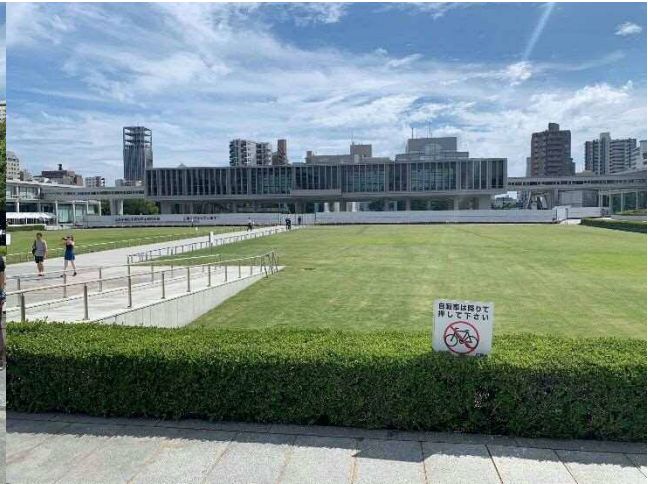
Faculties were under the earthquake proofing works
