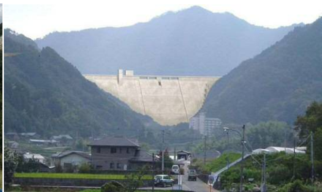
The Kabagawa Dam
