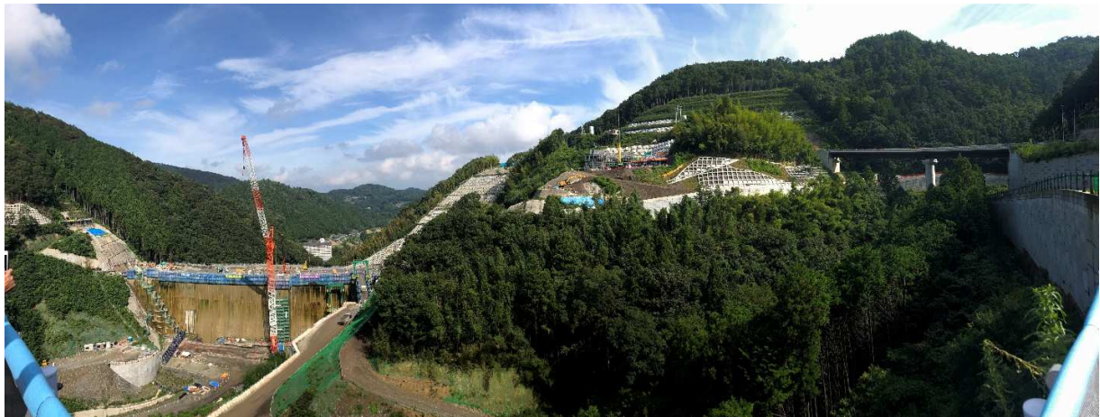
Figure 12. Kabagawa Dam Construction Site, Takamatsu, Nagawa
