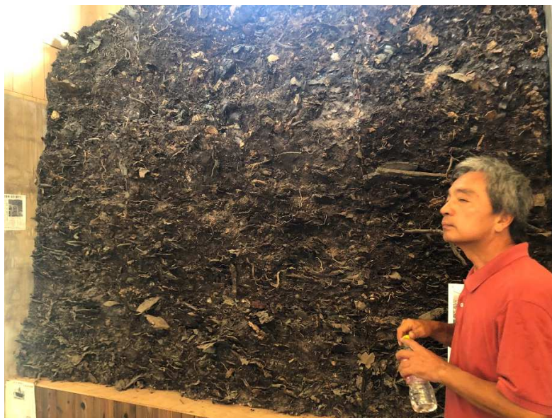
Figure 9. A fraction of the wall made from dumping waste
