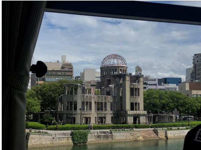
Figure 16. A dome damaged by the Atomic bomb
