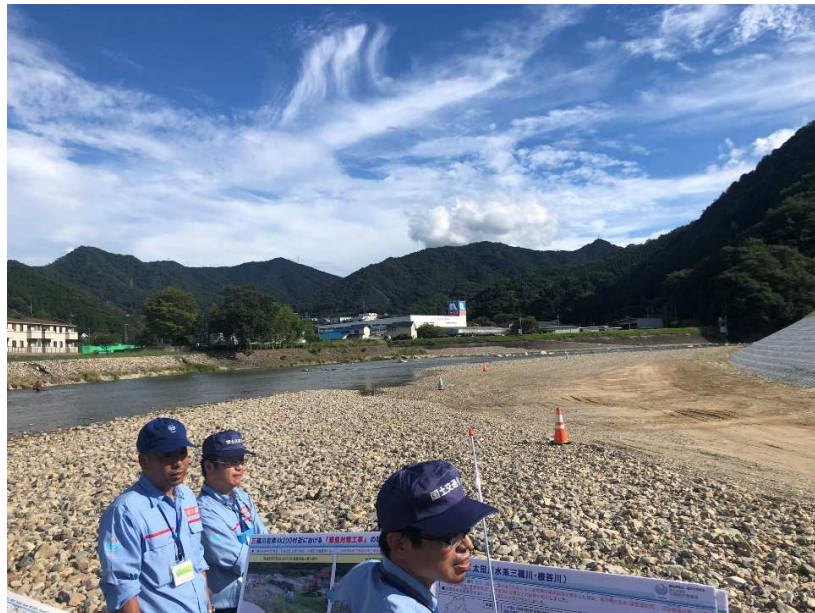
Figure 15. Misawa River damaged affected areas
