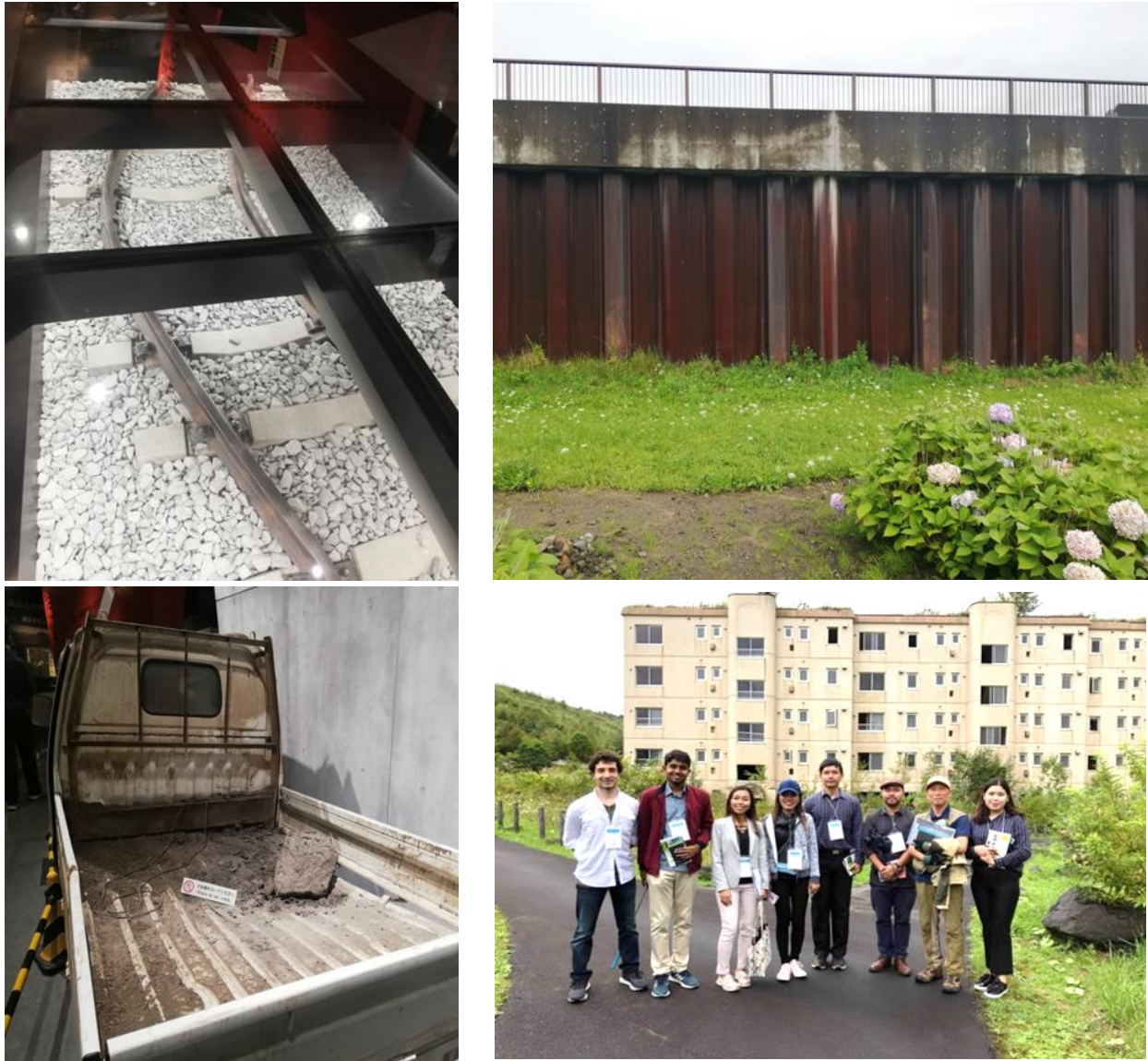
Figure 30: Affected railway track, vehicles and buildings due to Mt. Usu volcanic eruption and sheet pile to prevent mudslide from entering the locality in case of future calamities
