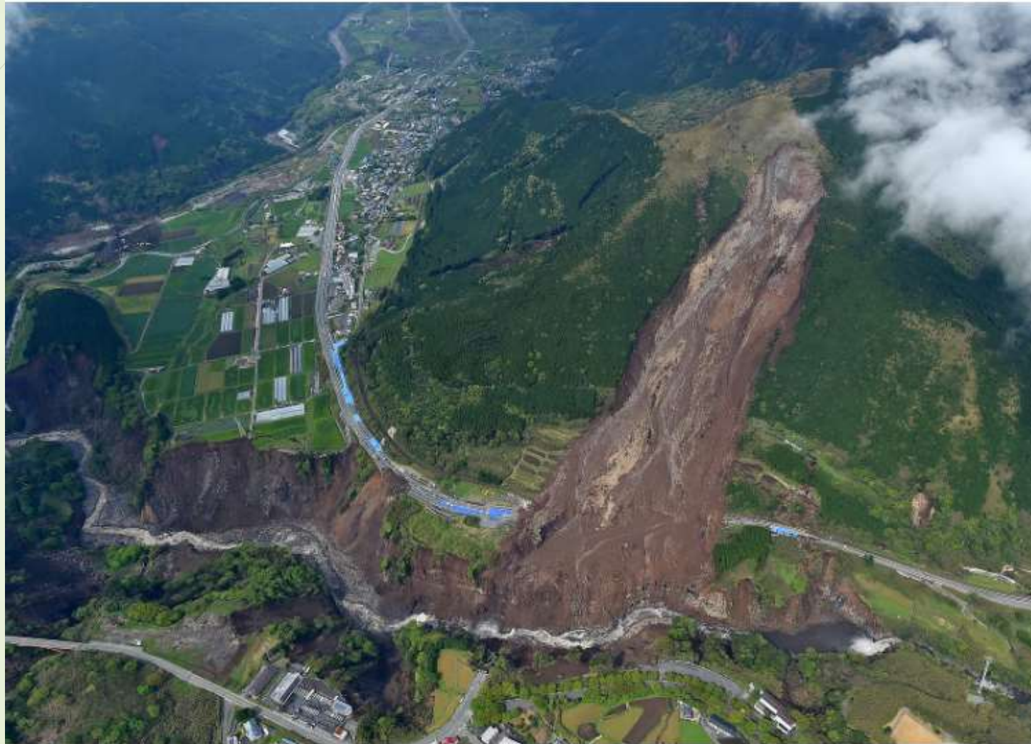
The Tateno district, background left, which was divided by the collapse of the Aso Ohashi bridge, is pictured in this photo taken from a Mainichi helicopter on April 22, 2016. (Mainichi)
