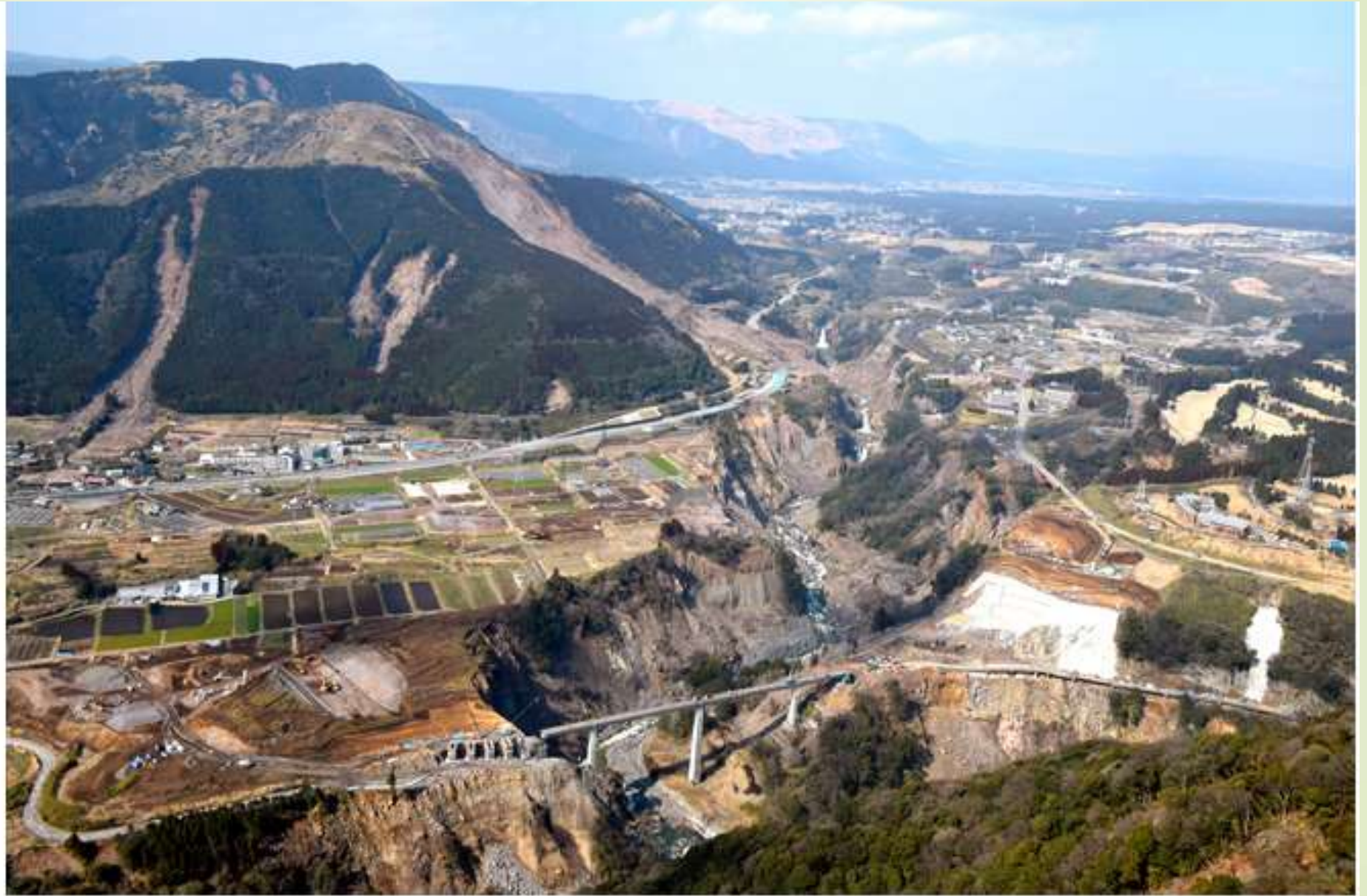
Aso-Choyo-ohashi bridge, foreground, is closed to traffic in Minami-Aso, Kumamoto Prefecture, on March. 14. The new Aso-ohashi bridge is planned to be built in the background. (Motoki Nagasawa)
