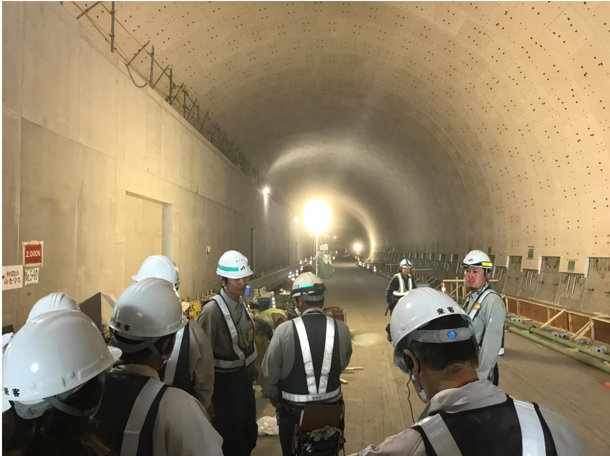
Figure 34 Shield Tunneling at Tajiri-Area Project
