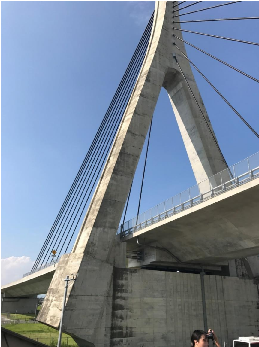
Figure 21 Yabegawa Bridge Cable
