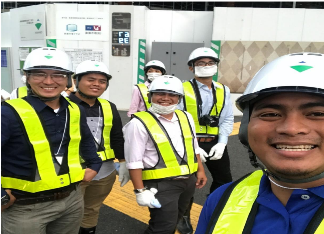
Figure 38 At Tokyo Railway Station Site
