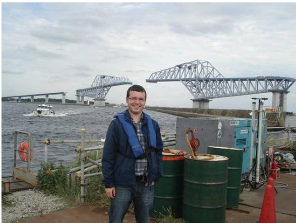
In addition, we saw Tokyo Port Bridge. Tokyo Port Bridge is steel truss bridge which is 2933 meters long and 87.7 meters high above water level. The architecture of this bridge was great. Earthquake resistance of the bridge was also unusual for our country. Arakawa Museum of Aqua one of the biggest rivers in Tokyo and we had chance to get some information about
