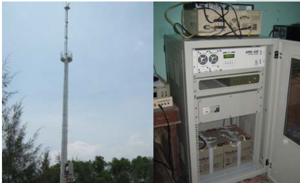
Project of Tsunami Warning System in high-risk areas 10 pilot tsunami warning in Da Nang city already setup
