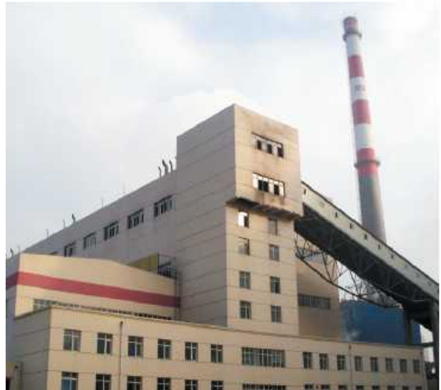
Photo 7 Power generation and central heat supply plant (front view)
