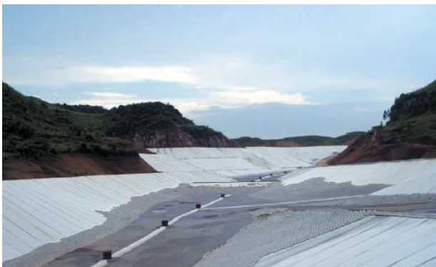
Photo 4 Garbage landfill under construction in mountainous area (Guangxi Zhuang Autonomous Region)
