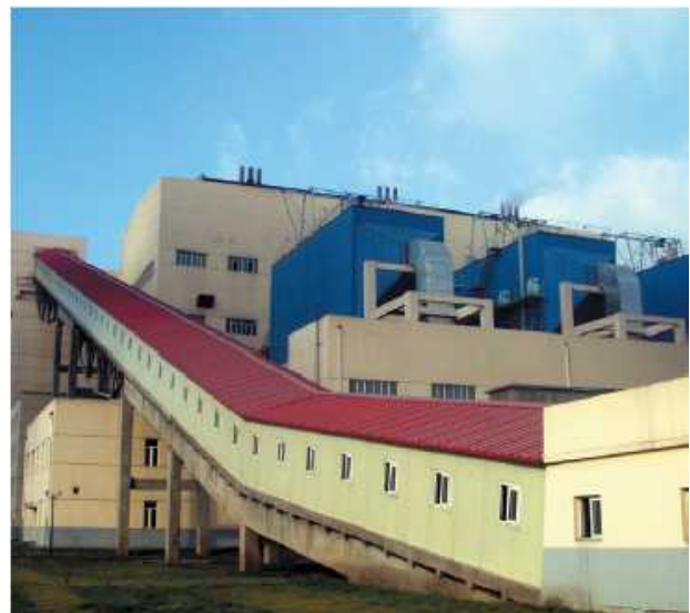
Photo 8 Same plant (rear view: coal conveyor)
